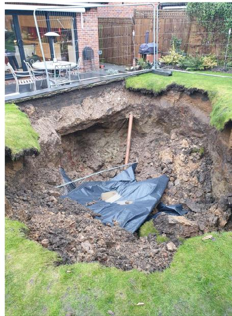
Loose debris was removed and the hole was backfilled with concrete.
