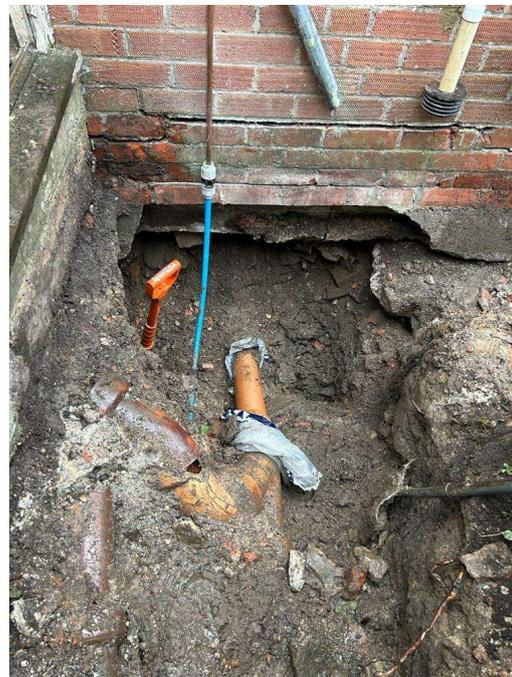
*Subsidence damage (brown arrow) to the brickwork above the leaking drain (red arrow).*
