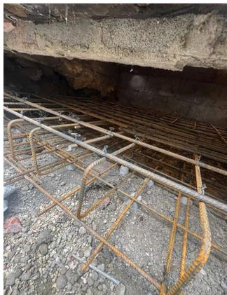
Allan designed a reinforced pad (left) to span the relatively short distance, spreading the load across adjoining walls.
